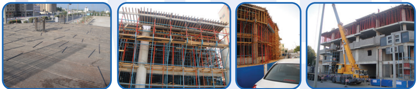
Scaffolding System & Shuttering for Slab
