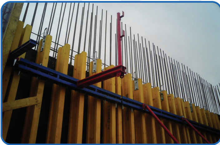
Retaining Wall Forms
