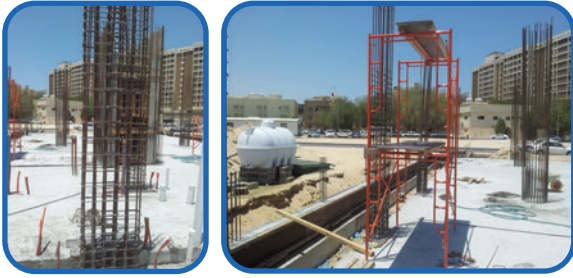
Concrete Column with Steel Reinforcement
