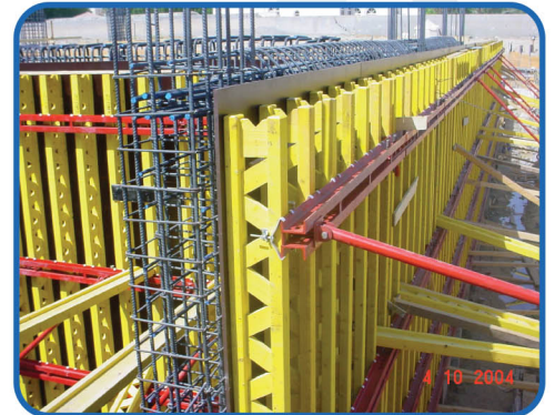
Retaining wall Forms
