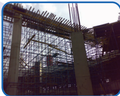
Scaffolding used in Damamm Tower.
