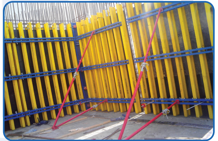
Retaining Wall Forms
