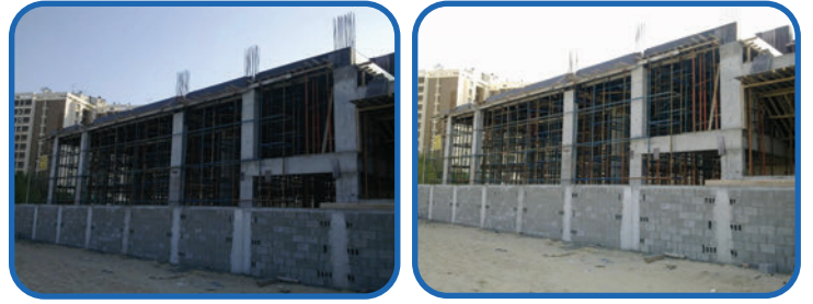
Scaffolding work used o support during the building process.
