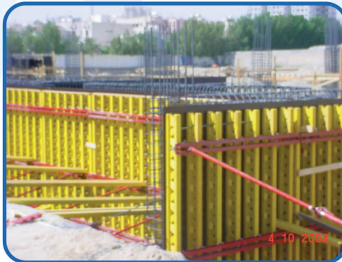
Retaining wall Forms
